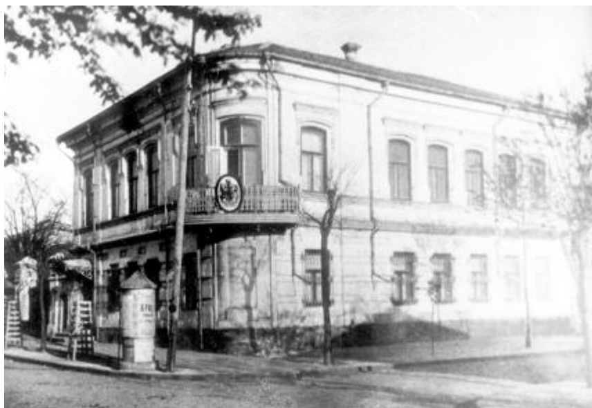
59. The building of the plant management
